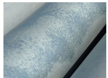
Figure 12: Mottled appearance of a newly galvanized pipe
