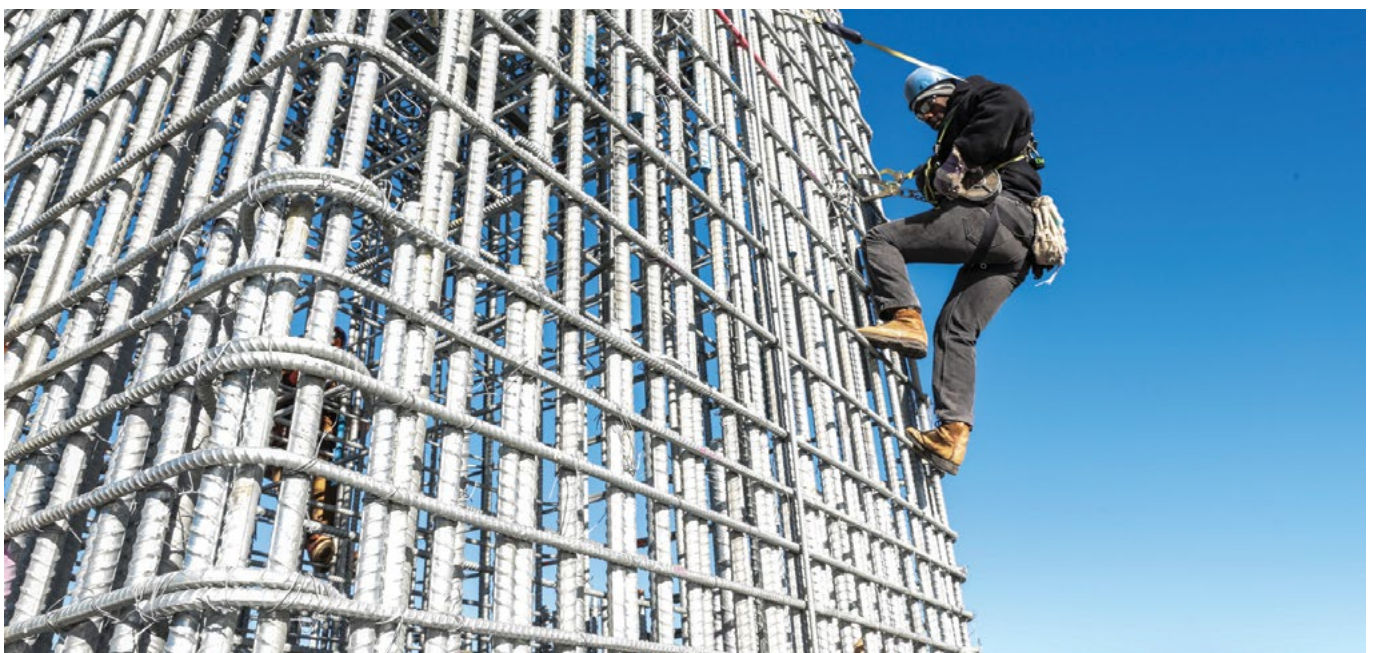
Field Handling Galvanized Rebar. (Photo Credit: New York State Thruway Authority)
