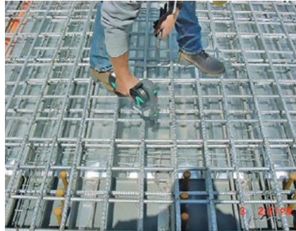
A galvanized reinforced deck being tied together with galvanized tie wire
