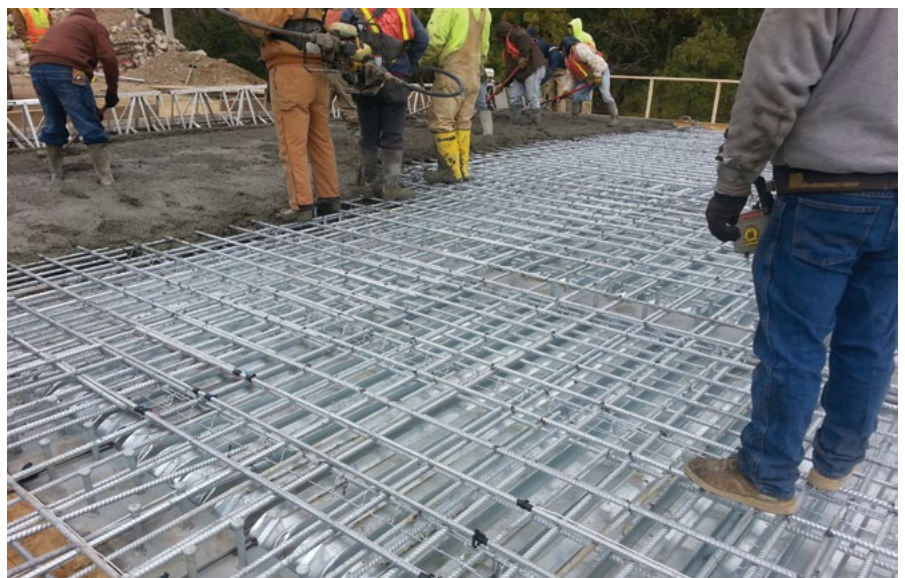
Installation of galvanized reinforcement on a bridge deck in the USA
