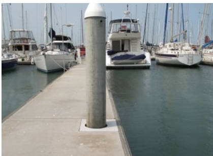
The floating pontoons at this marina at Sandringham, Victoria used galvanized reinforcement
