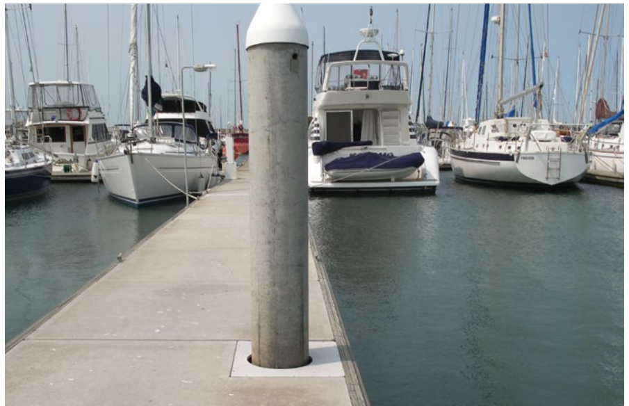
The floating pontoons at this marina at Sandringham, Victoria used galvanized reinforcement
