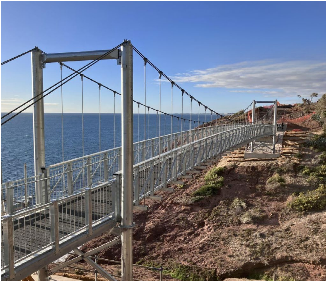
This cable suspension footbridge at Hallett Cove, South Australia makes extensive use of hot dip galvanized steel in a C5 location.
