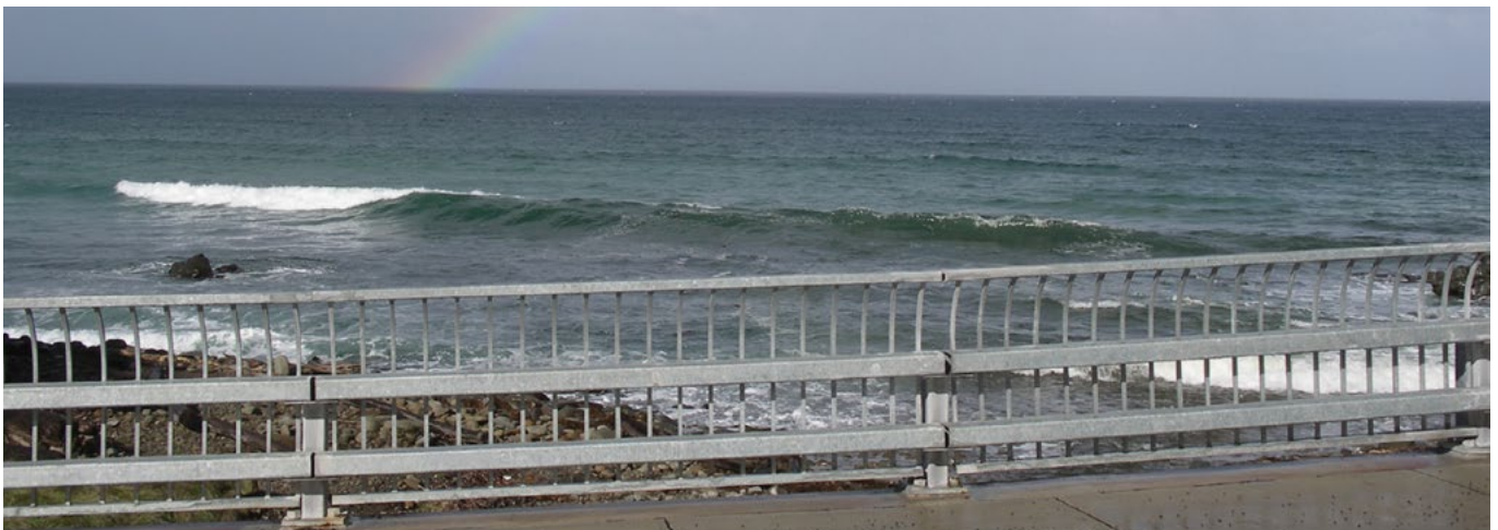
Galvanized guard rails have a good record of performance along the Great Ocean Road in Victoria.
