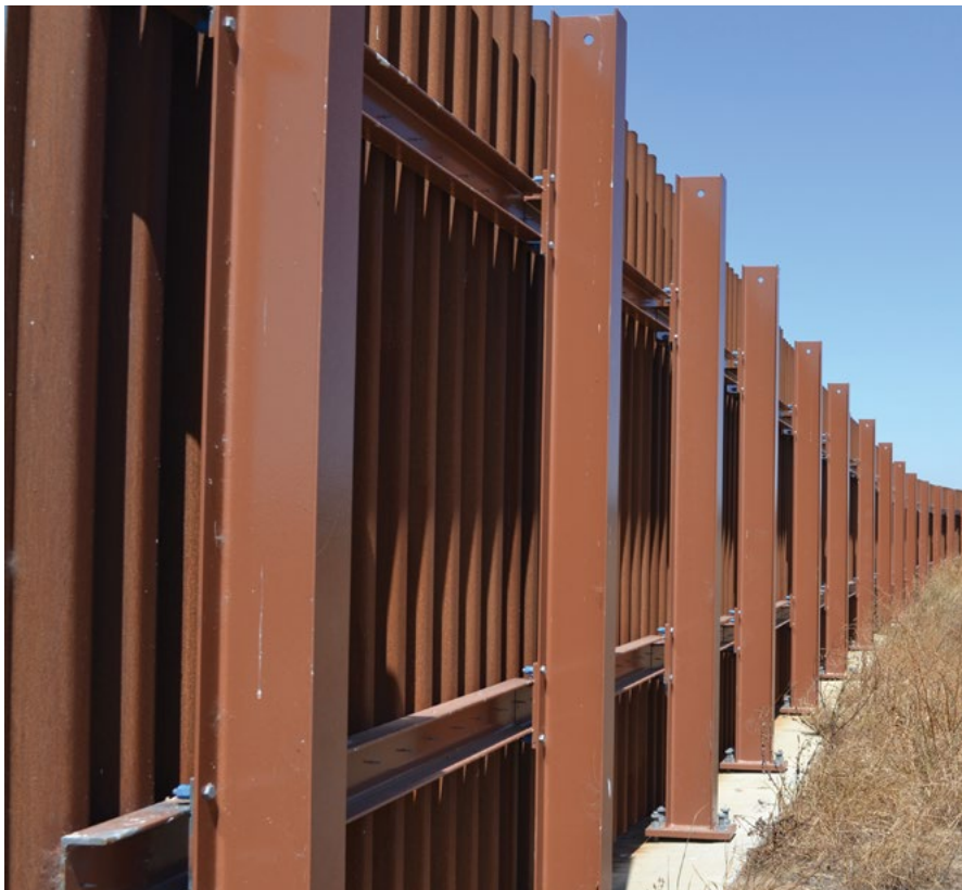
Baanip Boulevard Noise Wall Grovedale.
