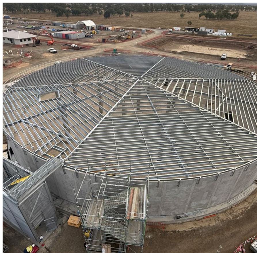
Tier 1 reservoir project in Queensland. Photo courtesy of NEACH
