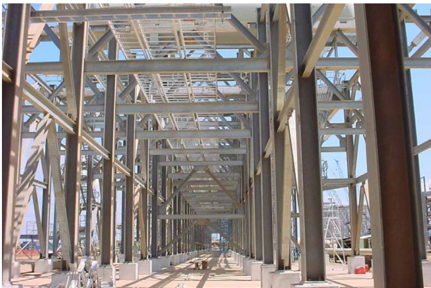
This gas processing facility in the NT is in a C3 coastal zone.
