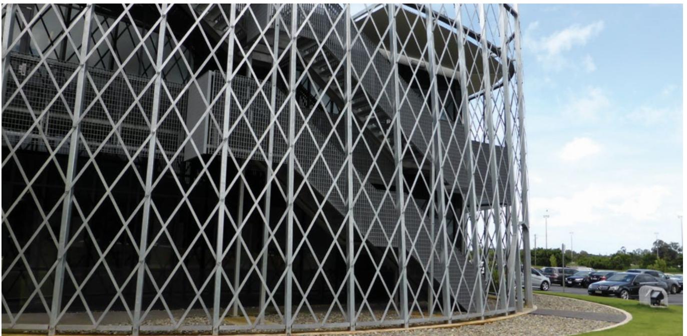
The Cairns Institute uses hot dip galvanized steel as a fabricated lattice facade.
