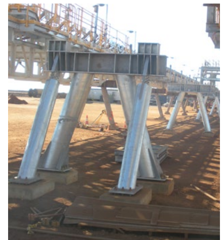
Galvanized conveyor frames are used successfully in the iron-ore mining industry
