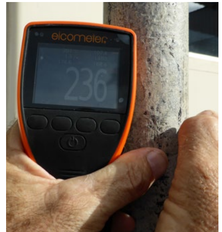
Many of the Morse Code line poles are still standing or have been recently recovered with near original coating thicknesses now at least 130 years on in a variety of severe exposure.
