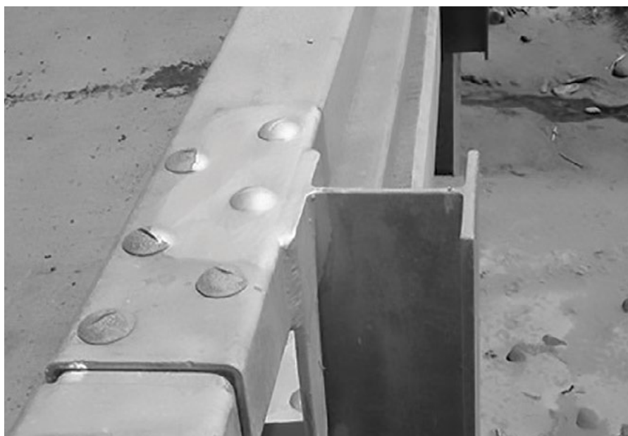
Figure 16: An example of a well repaired crash barrier in a severe marine environment
