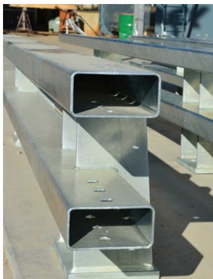
Figure 16: An example of a well repaired crash barrier in a severe marine environment
