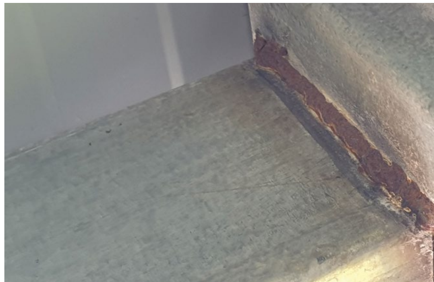
Figure 15: Badly repaired field welds which are corroding long before the rest of the fabrication
