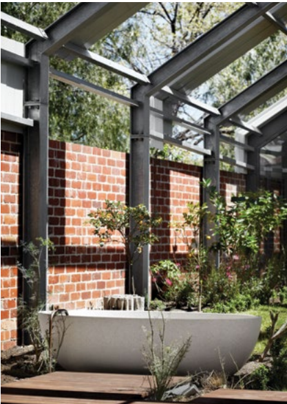
Figure 2: HDG fasteners are used in this domestic application to join both light steel purlins and structural columns to the portal frame (Cut Paw Paw by Andrew Maynard Architects, Photo by Tess Kelly)
