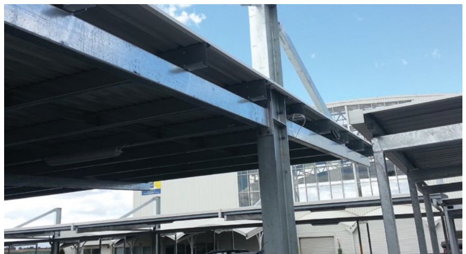
Figure 10: A car park structure with typical bolted connections
