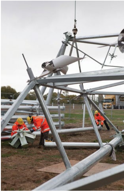
Figure 17: Modular construction is enabled through bolted connections
