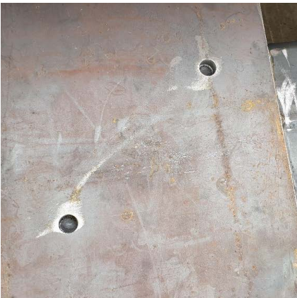
Figure 31: Overlapped surfaces larger than 10,000 mm 2 require venting.
